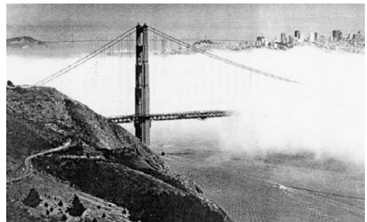
Fog rolling in under the Golden Gate Bridge.
